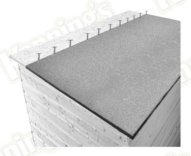
For the next piece of felt, repeat the process but from the front edge this time. This piece will over lap the part you installed previously to give you a fully covered roof, again secure in place using 20mm Clout Nails (FIX 3), spaced approx. 100mm apart.
